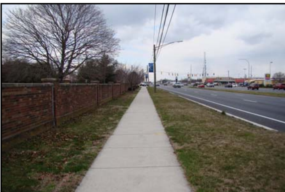
DSU Sidewalk (existing)
