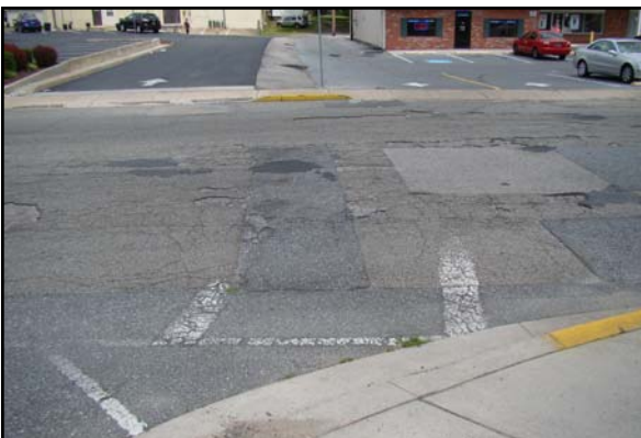
Existing Crosswalk (Looking East)
