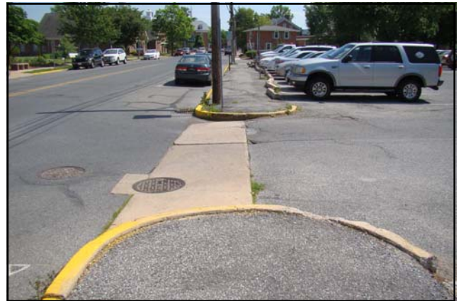
Kings Highway (Looking South)
