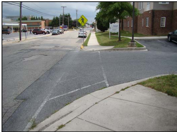
South New Street (Looking South)
