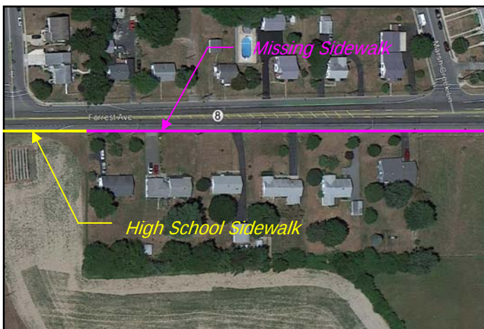
Route 8 (Adjacent to Dover High School)
